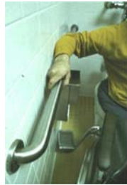
wall-mounted bar supports use and point loads
